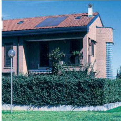
Example of sloped roof installation
