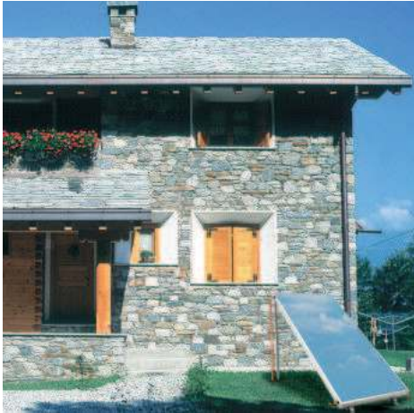
Example of ground installation
